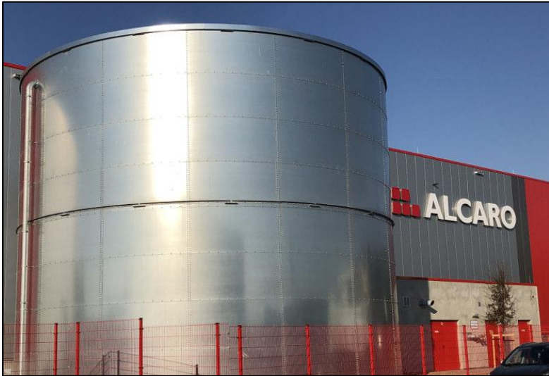
Sprinklertank 800 qbm
