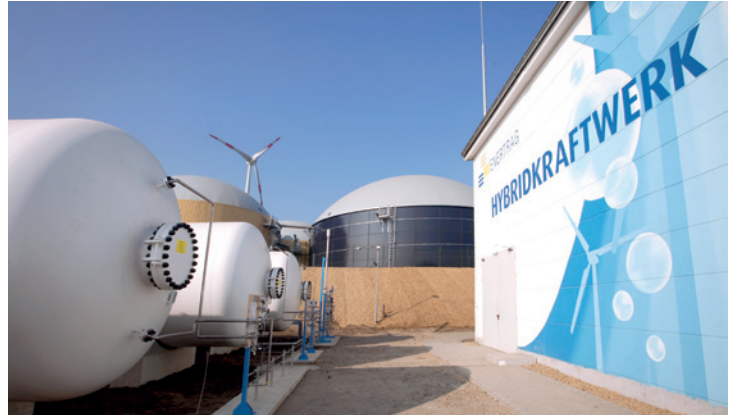
The ENERTRAG hybrid power plant in Prenzlau
